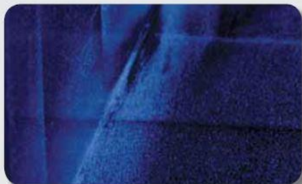
picture 17 detail of the residual dirt highlighted by the Wood lamp in the proximity of the corner of the sheet metal duct
