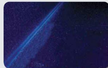
picture 13 detail of the residual dirt highlighted by the Wood lamp in the proximity of the corner of the P3ductal standard duct
